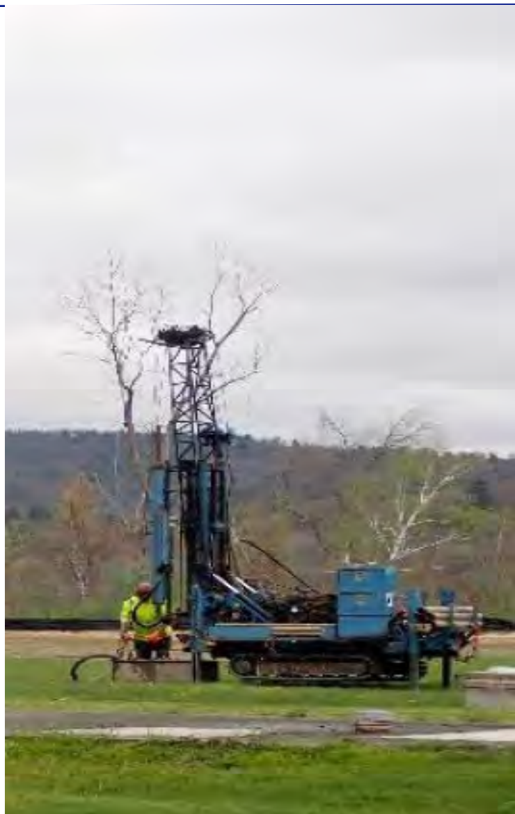
Adding Monitoring Well East of N Leach Field
