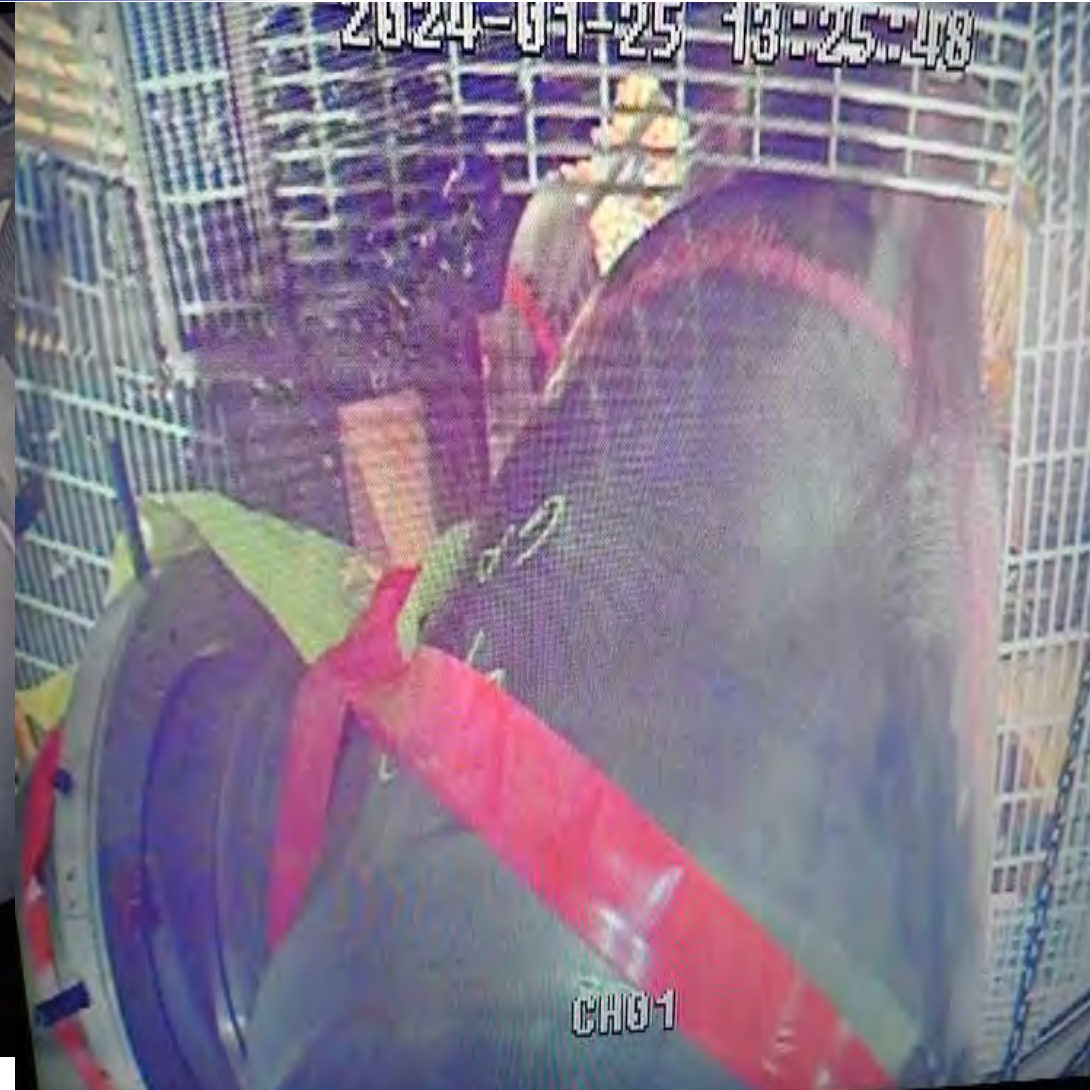
Rigging Out a Section of Cut Piping
