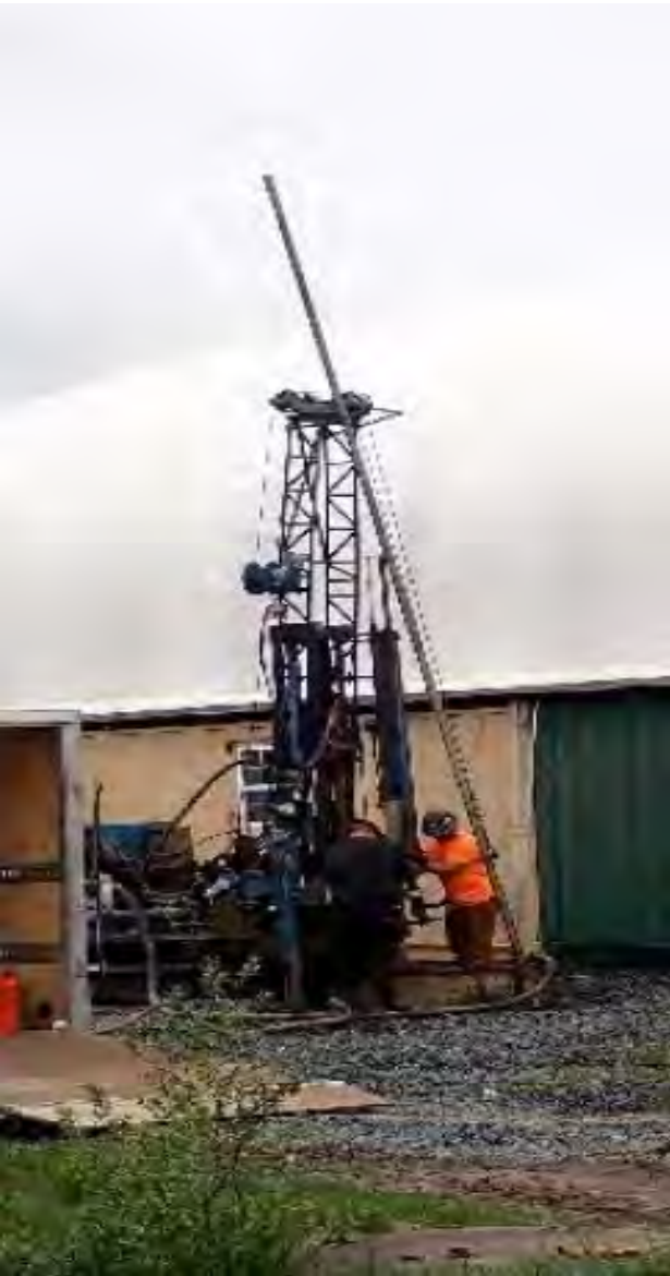
Adding Monitoring Well South of Plant Complex
